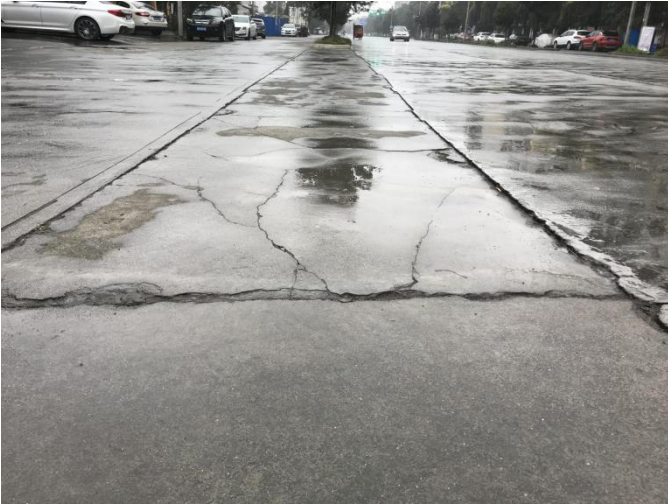
塘汛街道场镇塘汛街西段车行道现状
